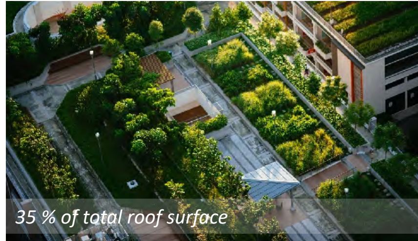
Intensive green roofs
